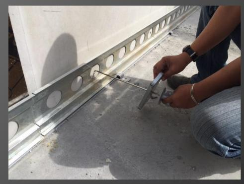
Once rail is installed and clipped down insert the first pin clamp with backing plate through the hole and out the other side.
