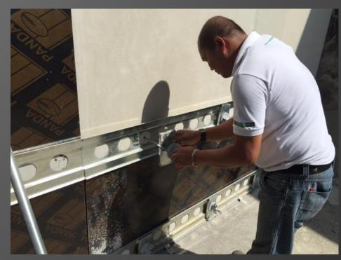
then install the other 3 pins and clamps tighten lightly before installing next plywood
