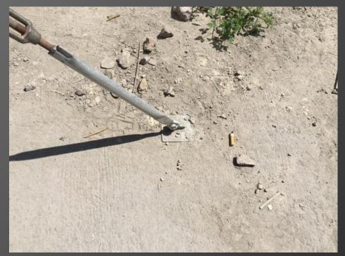
secure the brace pad to the concrete slab by either concrete nails or preferably reusable concrete screws
