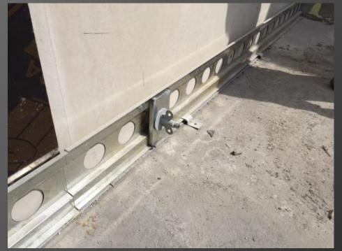
Once pin is inserted the worker on the other side of panel installes the pin lock clamp into the groove on the pin shaft and tightens it with the allen key wrench.
