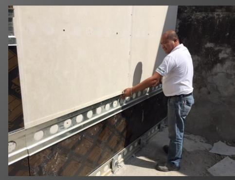
the next rail is placed and again using a drill, make holes though the centre of the rail hole to allow the pin to pass through the wall.
