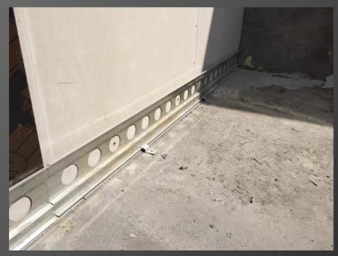
once panels installed and temp braced ( on rear side ) the first rail can be installed , it is secured down to the slab with rail clamps as shown , these are secured with concrete nails or preferably reusable concrete screws , once done a 10mm hole is drilled horizontally through the rail hole as shown , every 4<sup>th</sup> hole
