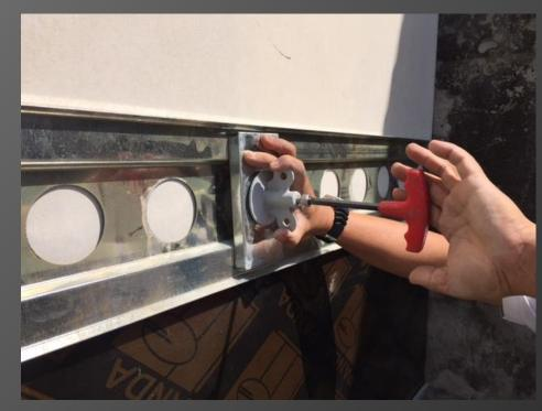
install the next rail and lightly tighten the first pin , once done install the balance three pins again lightly tighten prior to next plywood install
