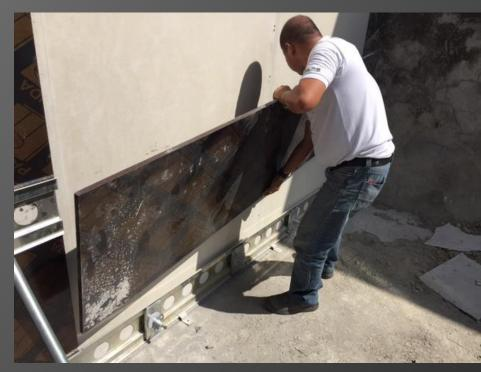
the installer can proceed with installing the first plywood 2 feet by 8 feet sheet
