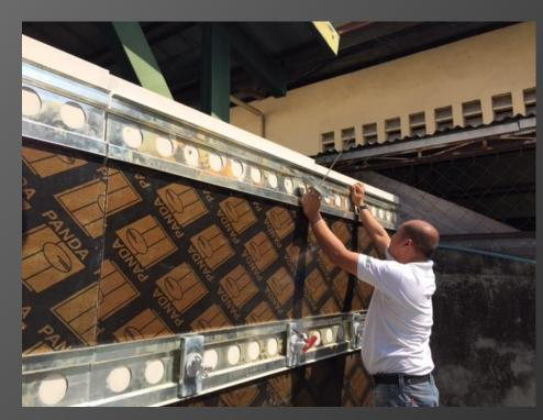
position the next rail , drill the holes for pins and insert first pin and lightly tighten to hold all in position
