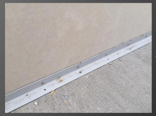
Plaswall panels are installed as per the normal procedure using reusable angles or bottom GI tracks concrete nailed or concrete bolted to slab this will keep panels aligned and by the use of temporary braces the panel is installed and plumbed vertical.
