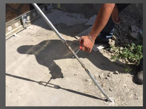
when secured the brace turnbuckle can be rotated to fine tune the vertical plumb of the wall, prior to this the temporary braces attached to the rear of the wall should be removed.
