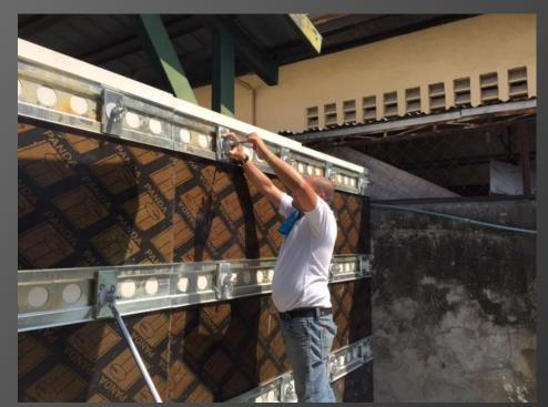
Then install the pin clamps and tighten
