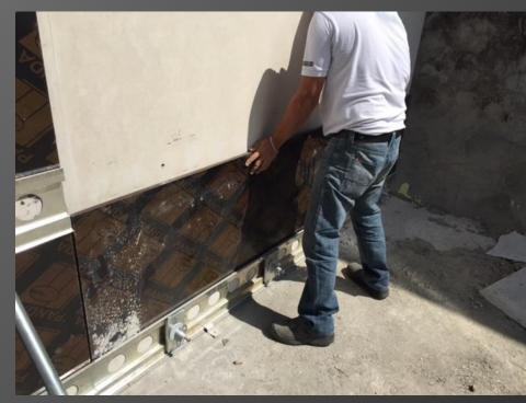
the plywood will slip easy into the rail and be held , once this is in place the bottom rail clamps can be tightened to hold the plywood firmly in position .
