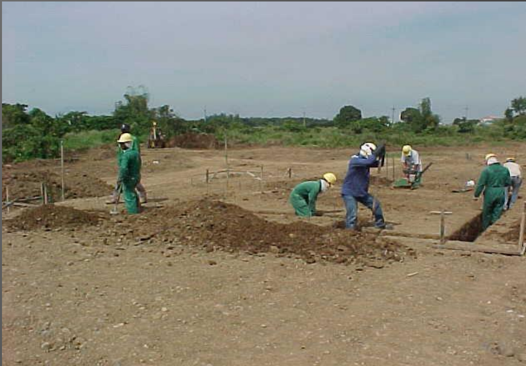
EXCAVATING FOR MAT FOOTING
