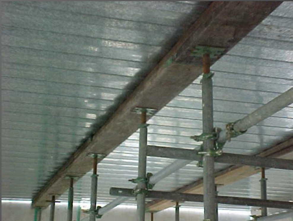
TYPICAL SETUP FOR STEEL DECK SLAB
